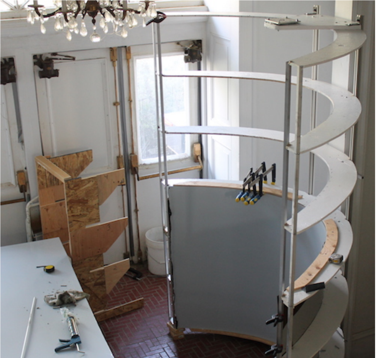
Attaching the first of two mirrors
